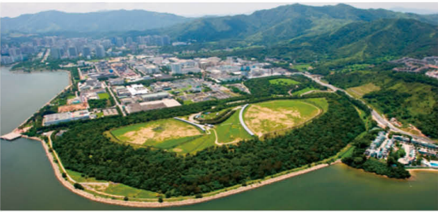
Aerial View of Hong Kong Tai Po Shuen Wan Landfill, 2022
