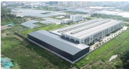
Bottom Ash Resource Utilization Treatment Workshop in Huangyan WtE Plant
