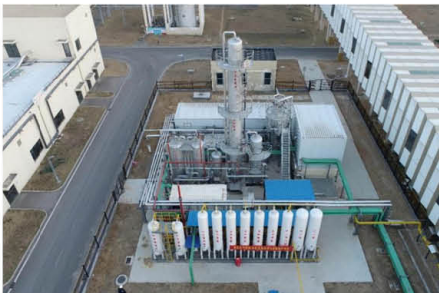
Qingdao West Coast Eco-Industrial Park Biogas Upgrading Project
