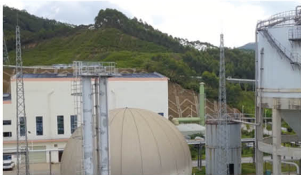
Wuzhou Eco-Industrial Park Food Waste Project
