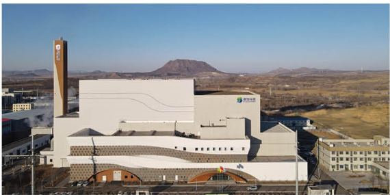
Chaoyang Industrial Steam Supply Plant
