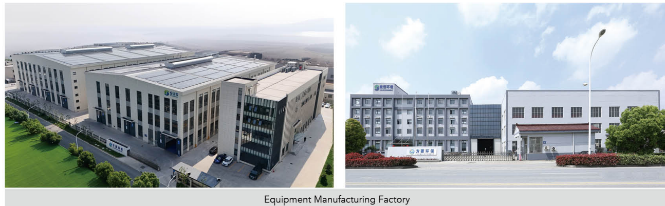
Equipment Manufacturing Factory
