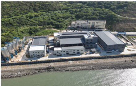
Fly Ash Resource Utilization Treatment Workshop Plant in Ningbo WtE Plant
